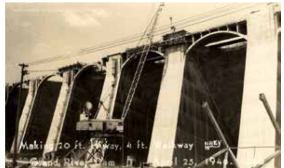
Pensacola Construction in 1940
